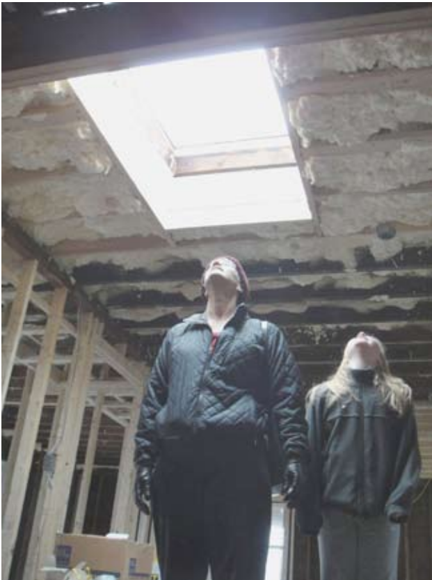
Left: Marin and Thea Clarkberg admire the second story skylight and the freshly sprayed-on foam insulation in the Third Street Meetinghouse.
